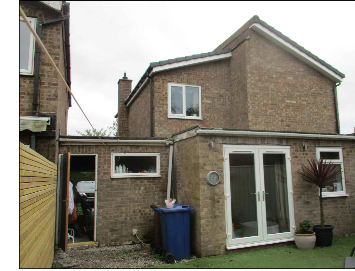
PHOTO IMAGE OF REAR ELEVATION (location of proposed infill Extension)
